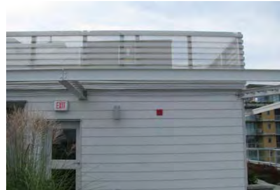
Architectural screening of rooftop mechanical equipment.
