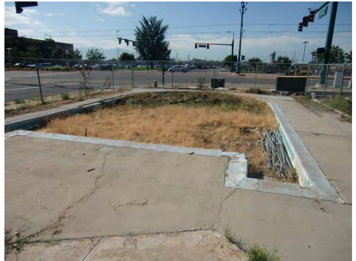
Photo 8. Former pool area
