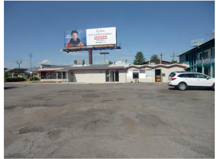
Photo 2. Subject property restaurant and office
