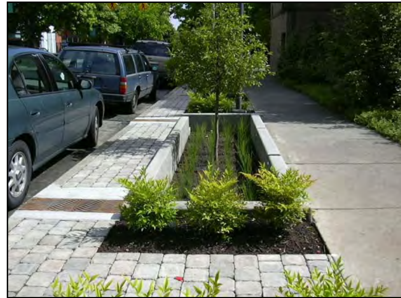
Streetscape with lid stormwater features integrated into landscaping design.
